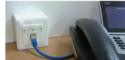
Example: Surface Mount Box Installation
