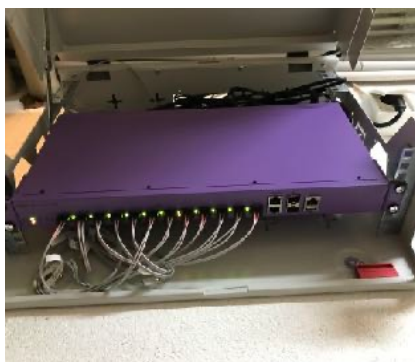
The gigabit POF-switches were placed according to constructional conditions and cabling.
