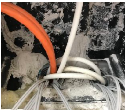
The POF cable was retrofitted and pulled into the existing cable-piping for electrical power, coaxial- and telephone-cable. No constructional intervention was needed.
