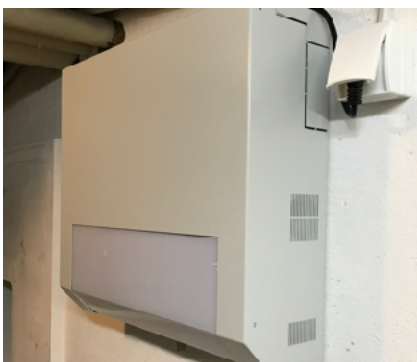
The gigabit POF-switches were placed according to constructional conditions and cabling.
